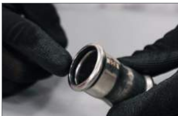
Controllo O-ring / Checking the sealing ring
